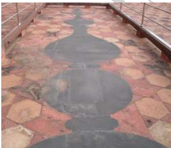
Fig: Finial floor tiling.
